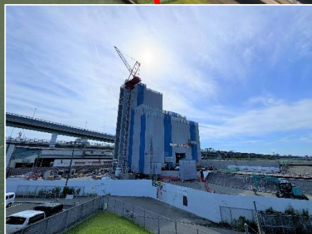
③換気所屋上階の構築
