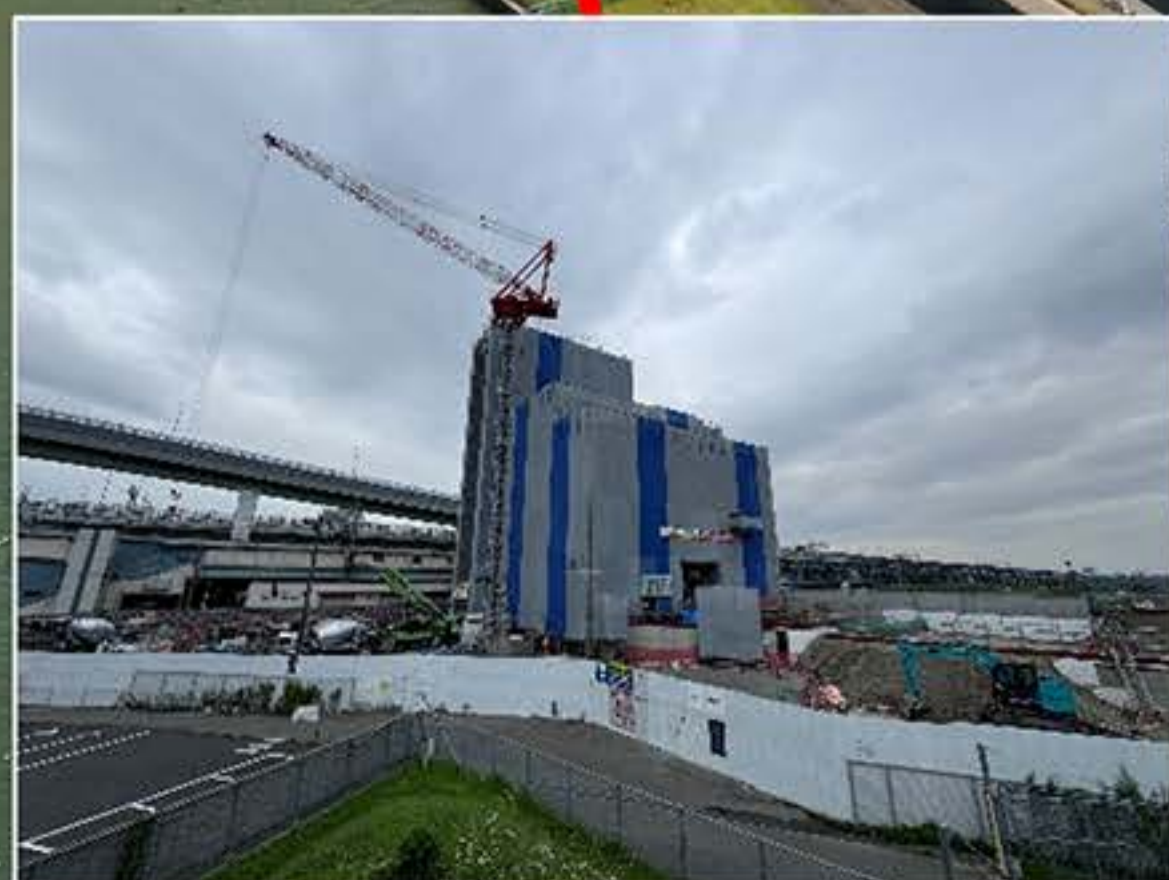
③換気所屋上階の構築
