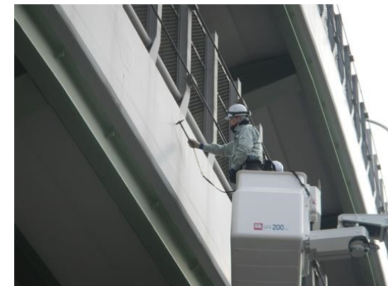
[橋梁点検状況]
